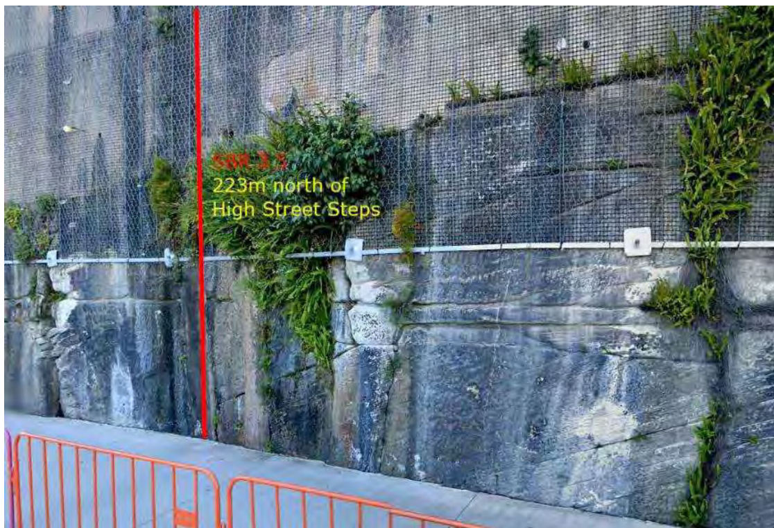
Figure 6: Location of downpipe SBR 3.5.
