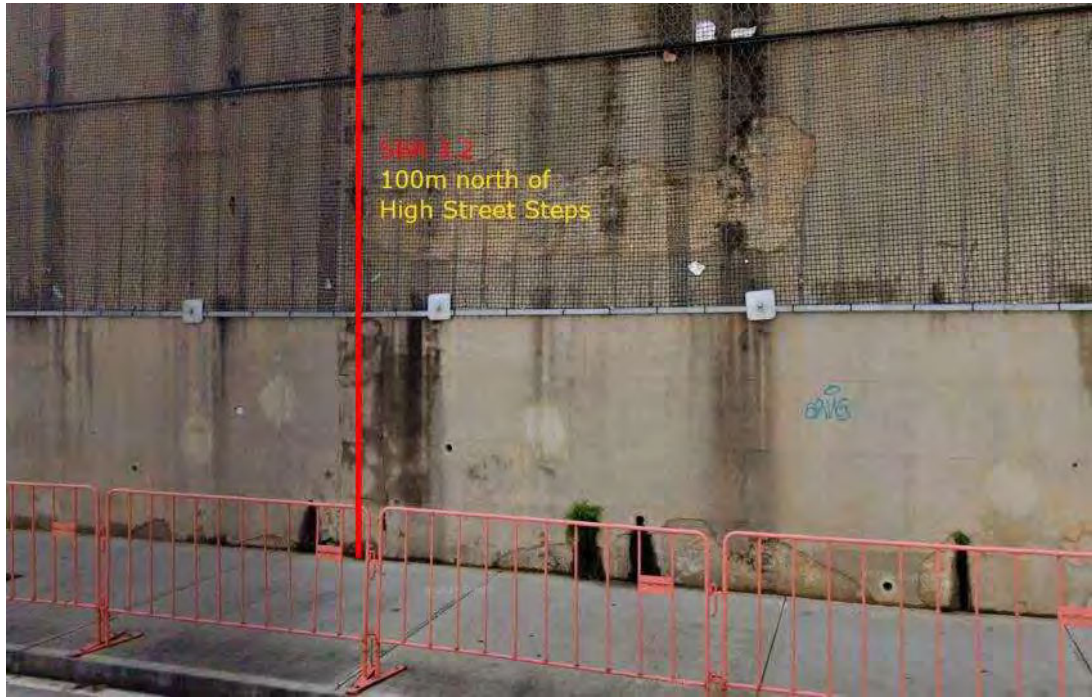
Figure 3: Location of downpipe SBR 3.2.
