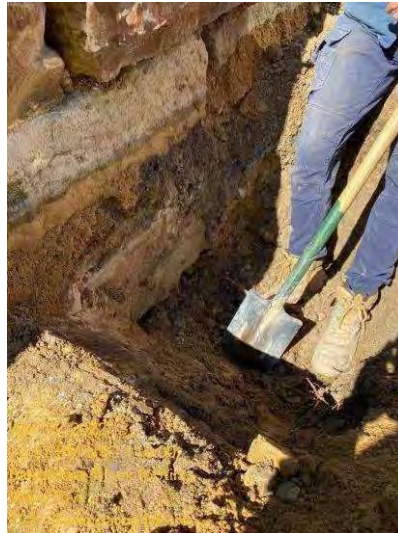
Figure 4: Concrete footing beneath sandstone blocks
