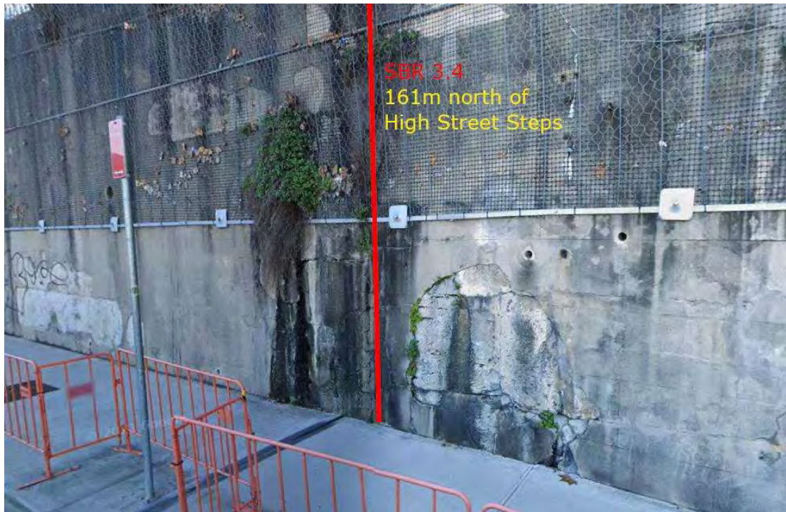
Figure 5: location of downpipe SBR 3.4.
