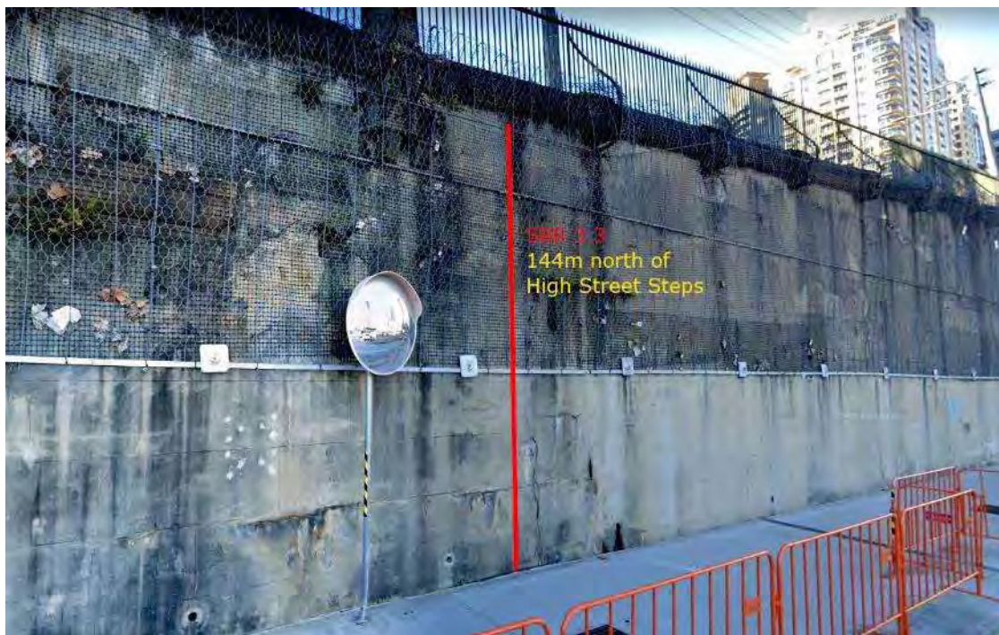
Figure 4: Location of downpipe SBR 3.3.
