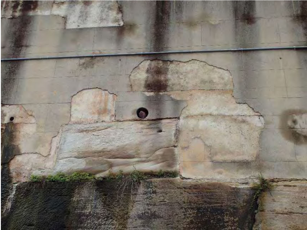
Figure 11: A section of the cutting and wall. The render is scored to replicate masonry blocks and is aligned along the line of the natural bedrock, above which the underlying sandstone blocks have been exposed.
