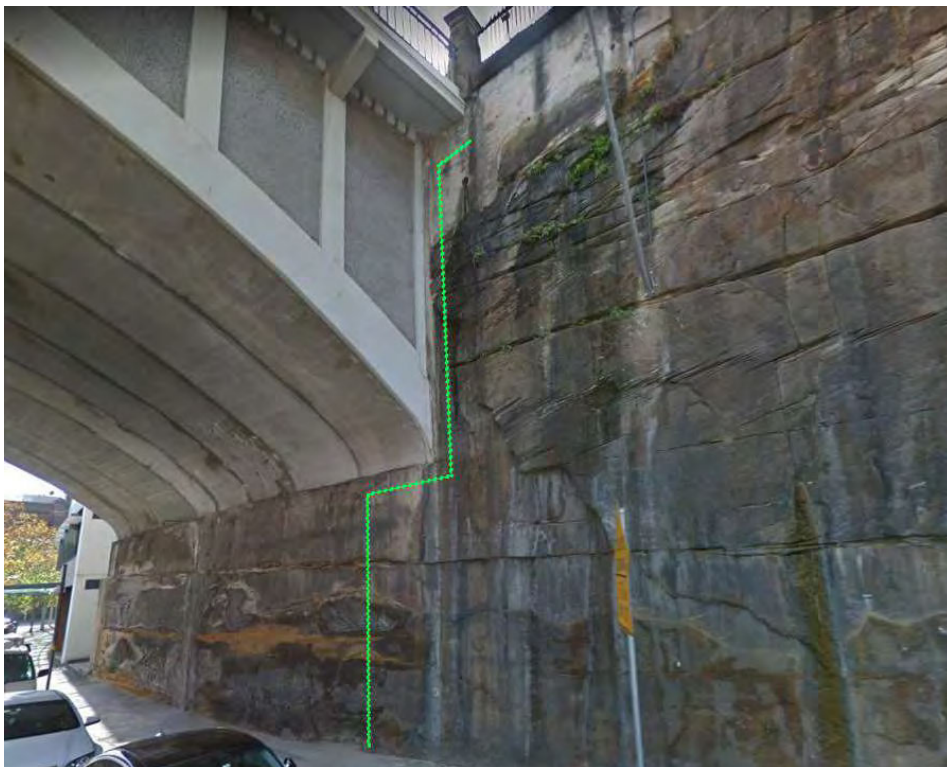
Figure 4: Proposed location of the gas diversion shown on a Google Street View capture taken in October 2014, before the acoustic shed was constructed. The Windmill Street bridge is at the left.
