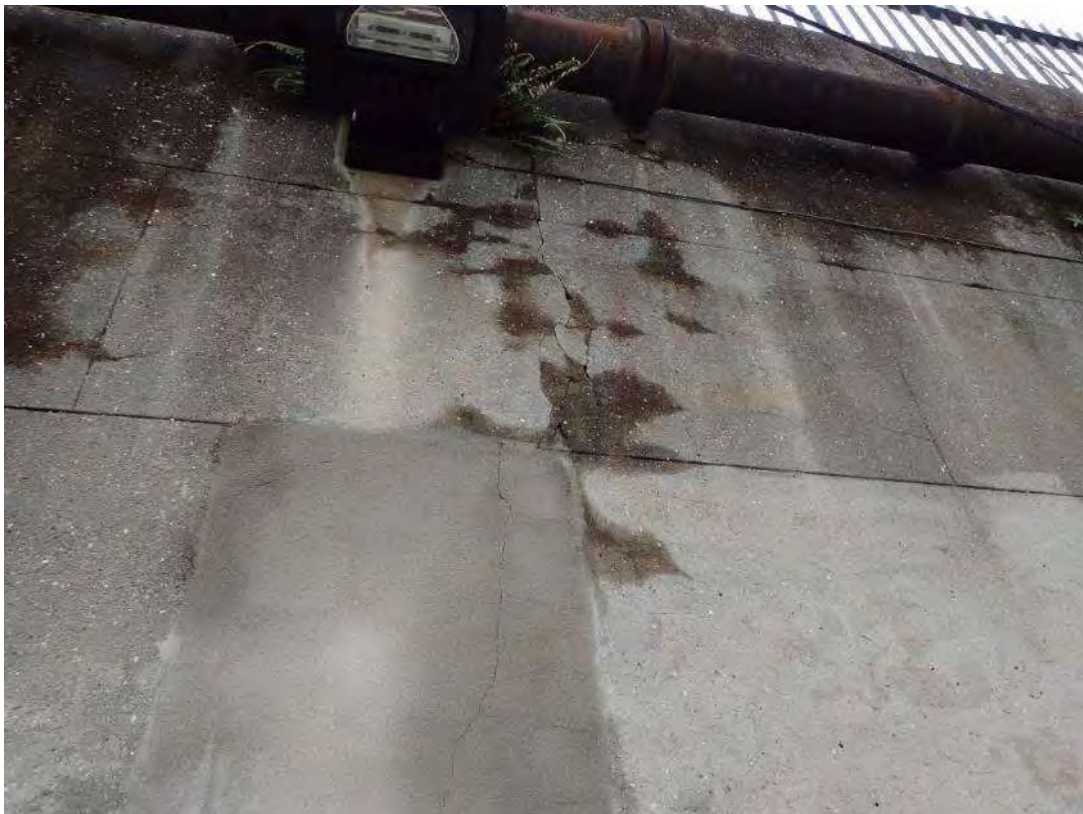
Figure 12: A patch of modern cement render surrounded by the original render. The white flecks are shell fragments.
