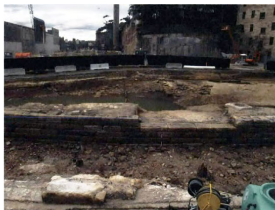
Figure 3.3: Dibbs' seawall looking northeast towards Dalgety stores (Austral Archaeology, 2016, p. 99)
